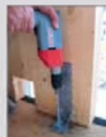
Fastening on wooden wall by means of fully threaded VGS screws (or, alternatively, with a loop nut)
