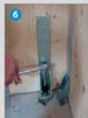
6 Nut positioning by means of suitable tightening torque
