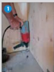
1 Concrete drilling and hole cleaning
