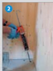
2 Injecting the vinyl ester chemical anchor in the hole
