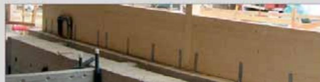
Positioning of the angle brackets on a concrete support typical for a wooden building
