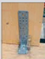
WHT installation and fastening to the wall by means of special screws
